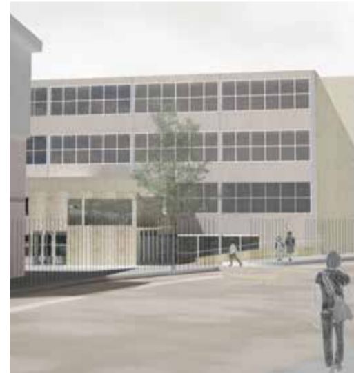
The new Entrance Building seen from Camden Road.
